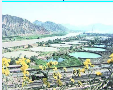
Modern water facilities
